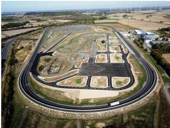
Figure 5. Aldenhoven Testing Center, Germany
