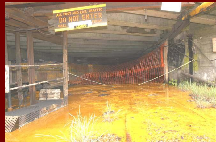
Abandoned mine portals
