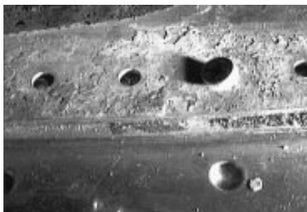
Fig 12a. surface with corrosion
